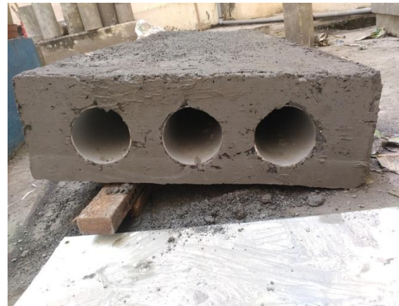
FIG 5.4 HOLLOW CORE SLAB AFTER CASTING
