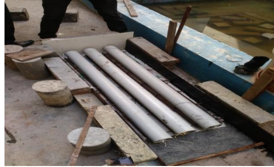
FIG 5.4 HOLLOW CORE SLAB BEFORE CASTING
